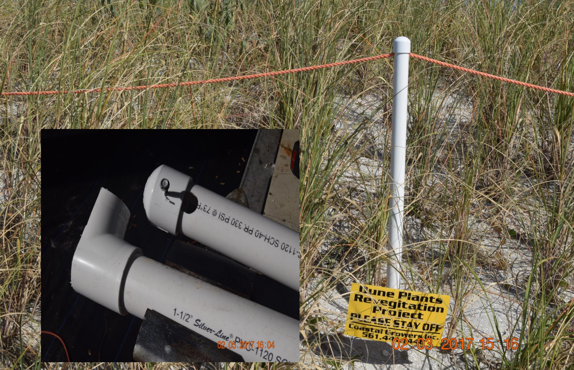
Low cost post and rope barrier, prefab 1.5 inch PVC with 3/8 inch polyethylene rope. About $1.50/foot installed.
