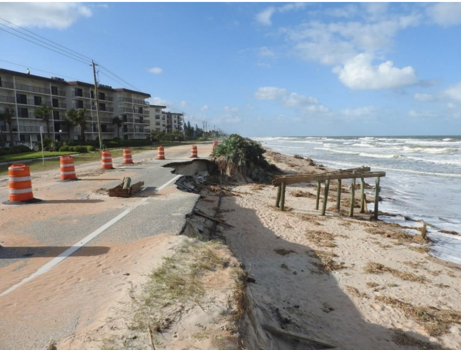
Ormond Beach State Road A1A Damage
