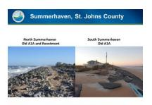
In southern St. Johns County along northern Summerhaven, the rock revetment that was constructed in the 1960's, was substantially damaged along with Old A1A. Also in south Summerhaven, Old A1A was substantially destroyed.
