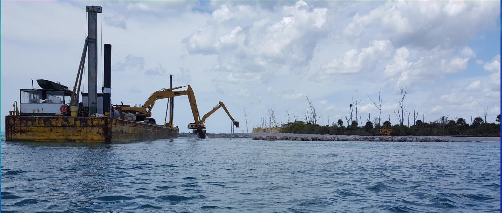
Excavating Next Section of Groin
