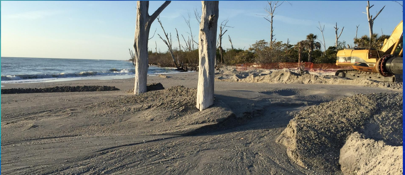
View looking North at Starting Point of Beach Fill
