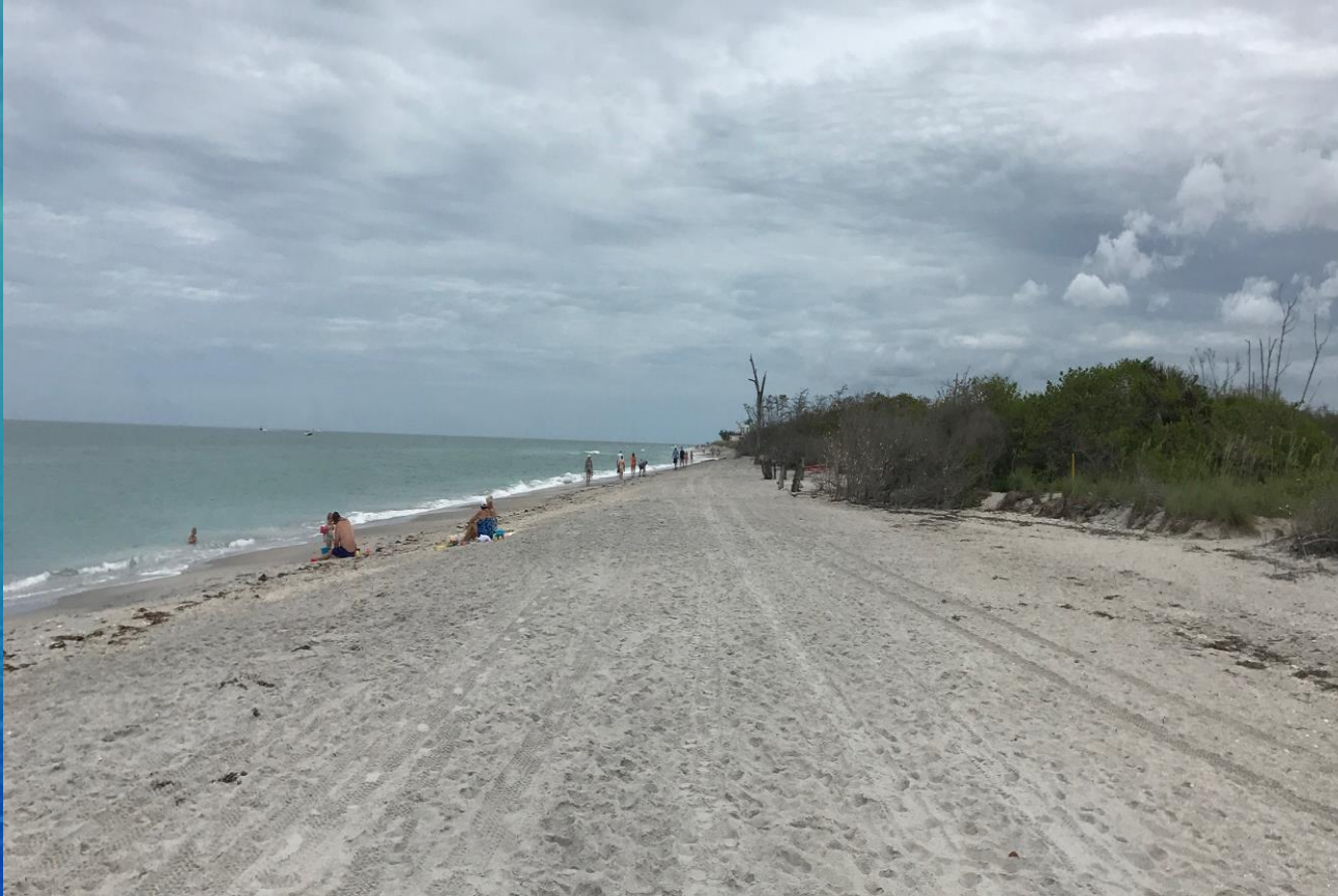
The New Beach Fill on Manasota Key (View North)
