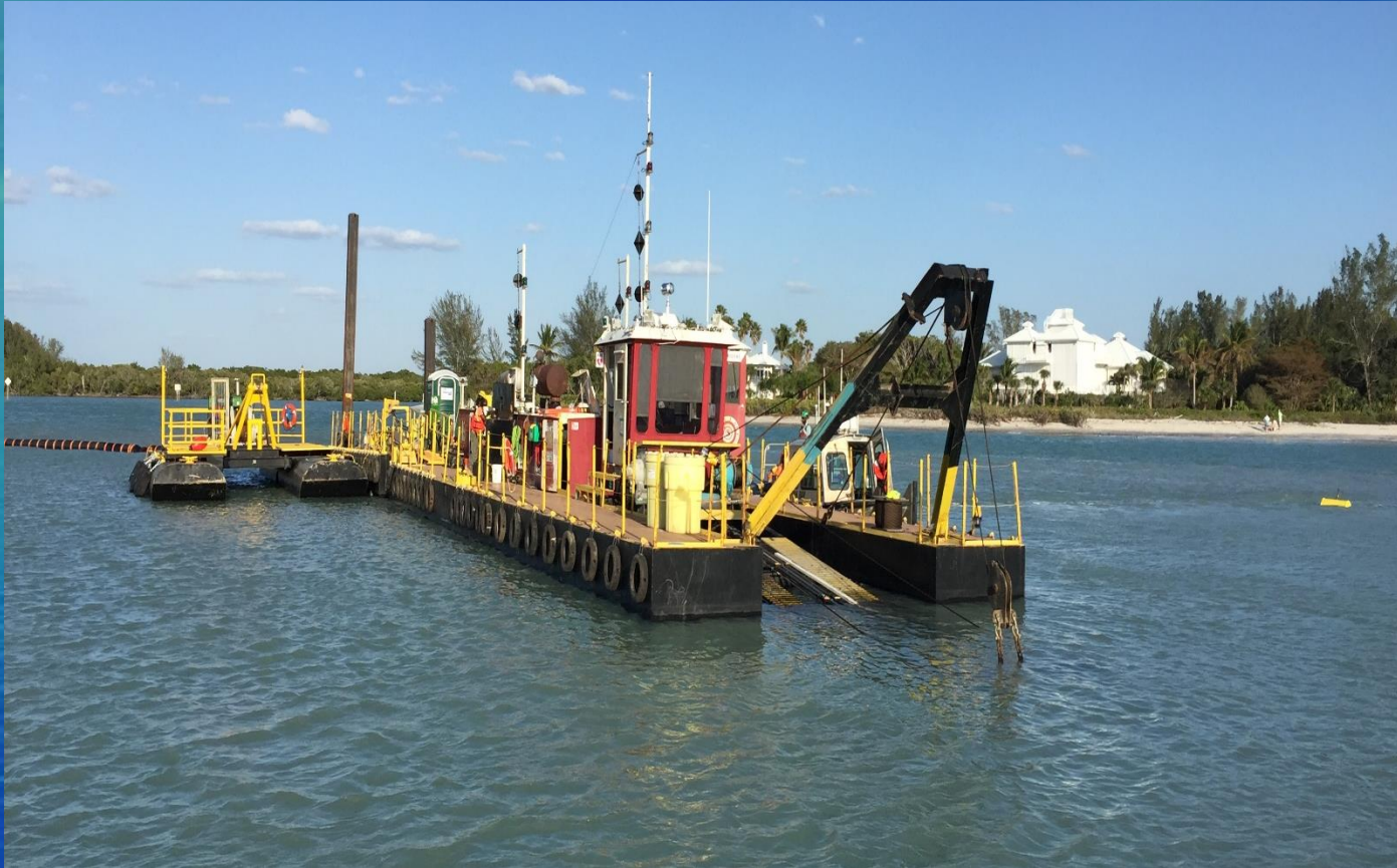
Great Lakes Dredge and Dock's Dredge 'Commodore'
