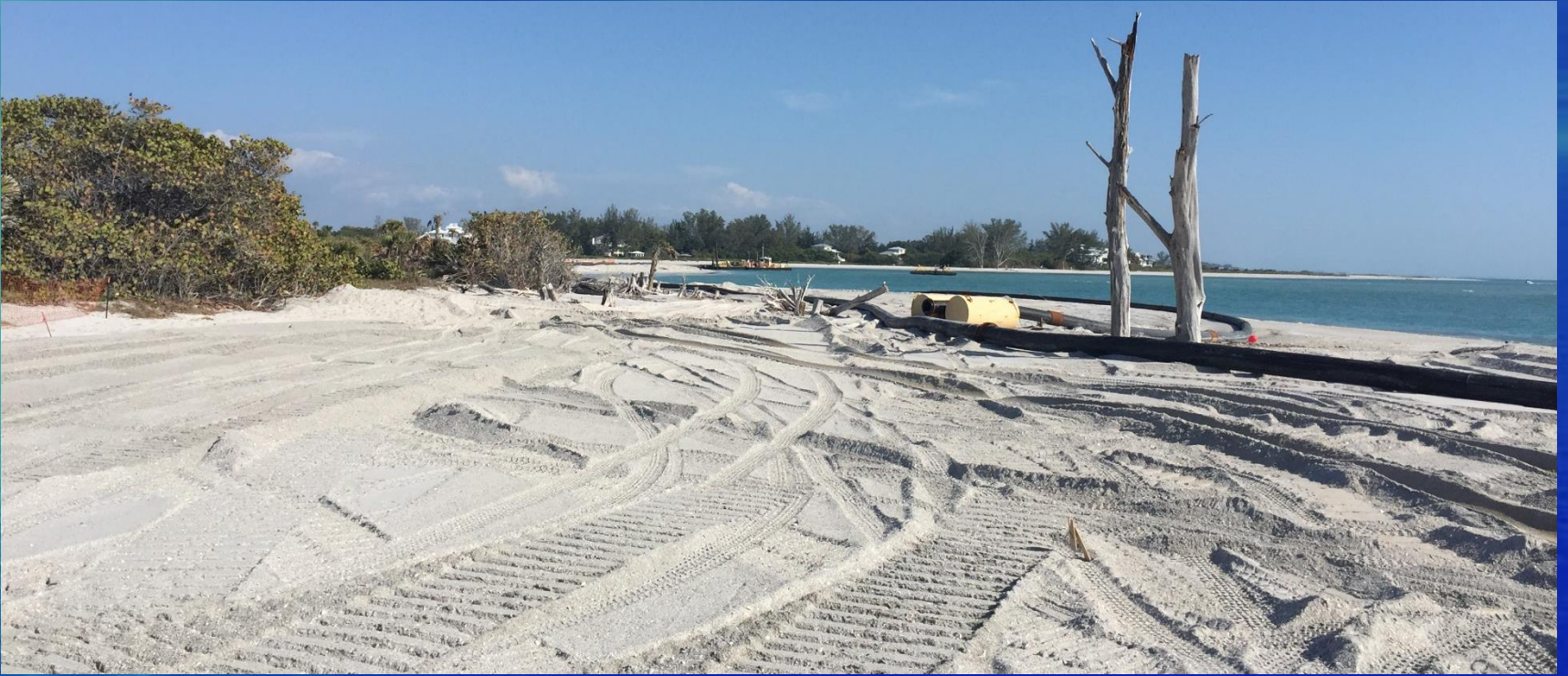
Beach fill looking South toward Stump Pass
