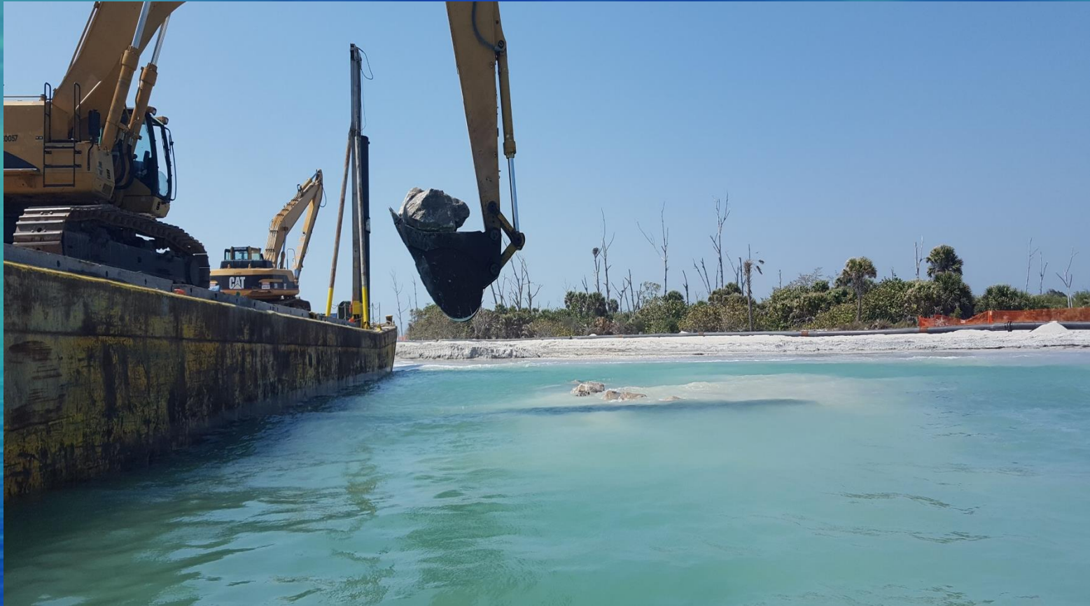
Armor Stone Being Placed on Groin
