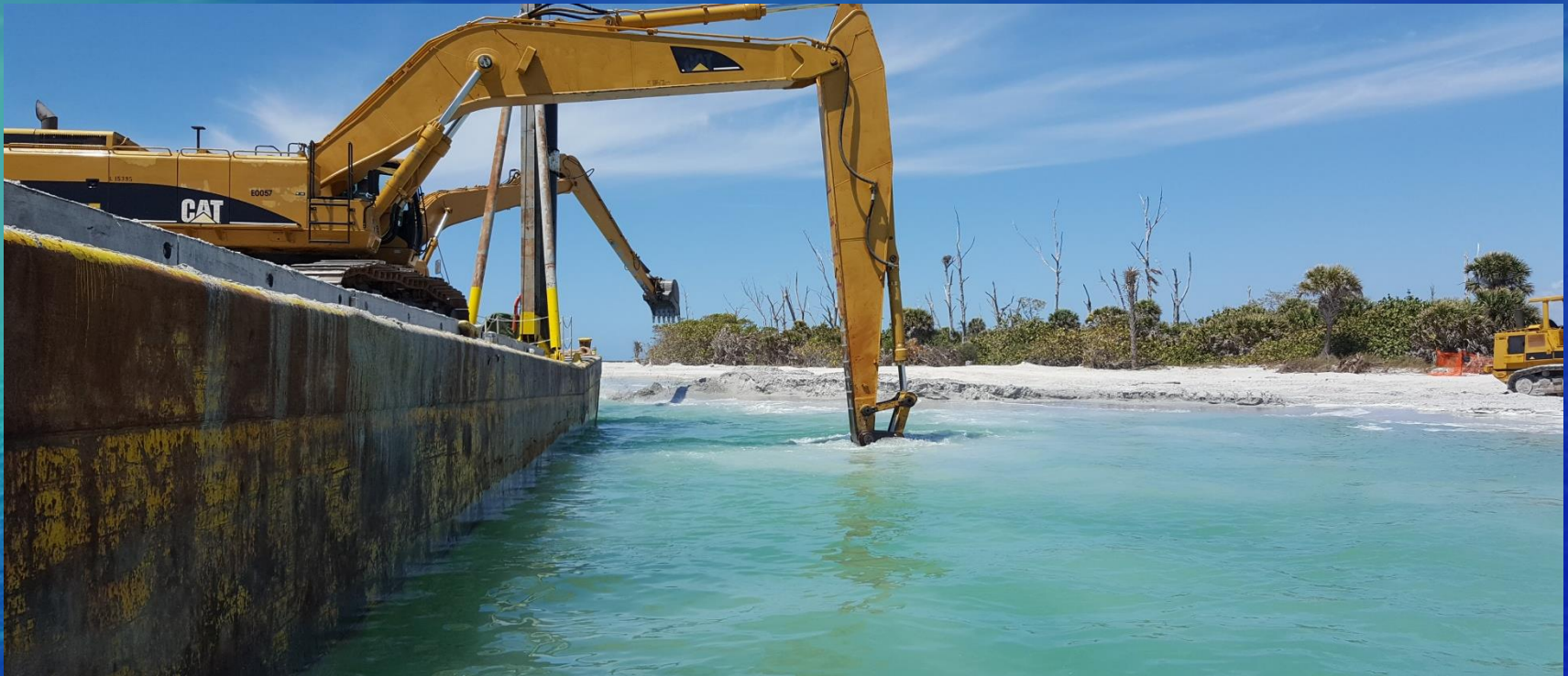
Excavating First Section of Terminal Groin
