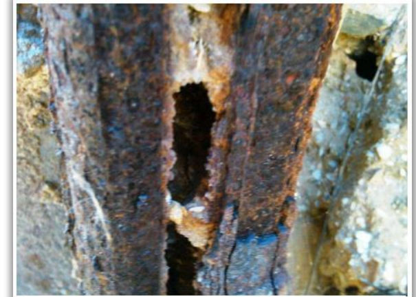
Figure 3 - Corrosion at the joint between two sheet piles showing complete section loss.
