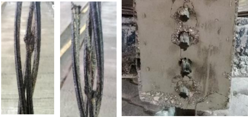
(a) & (b) CFRP strand failure during tensioning; (c) cracking following strands release.
