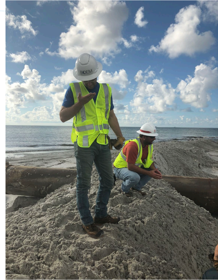
BOEM Staff Geologist inspecting newly placed OCS sand.
