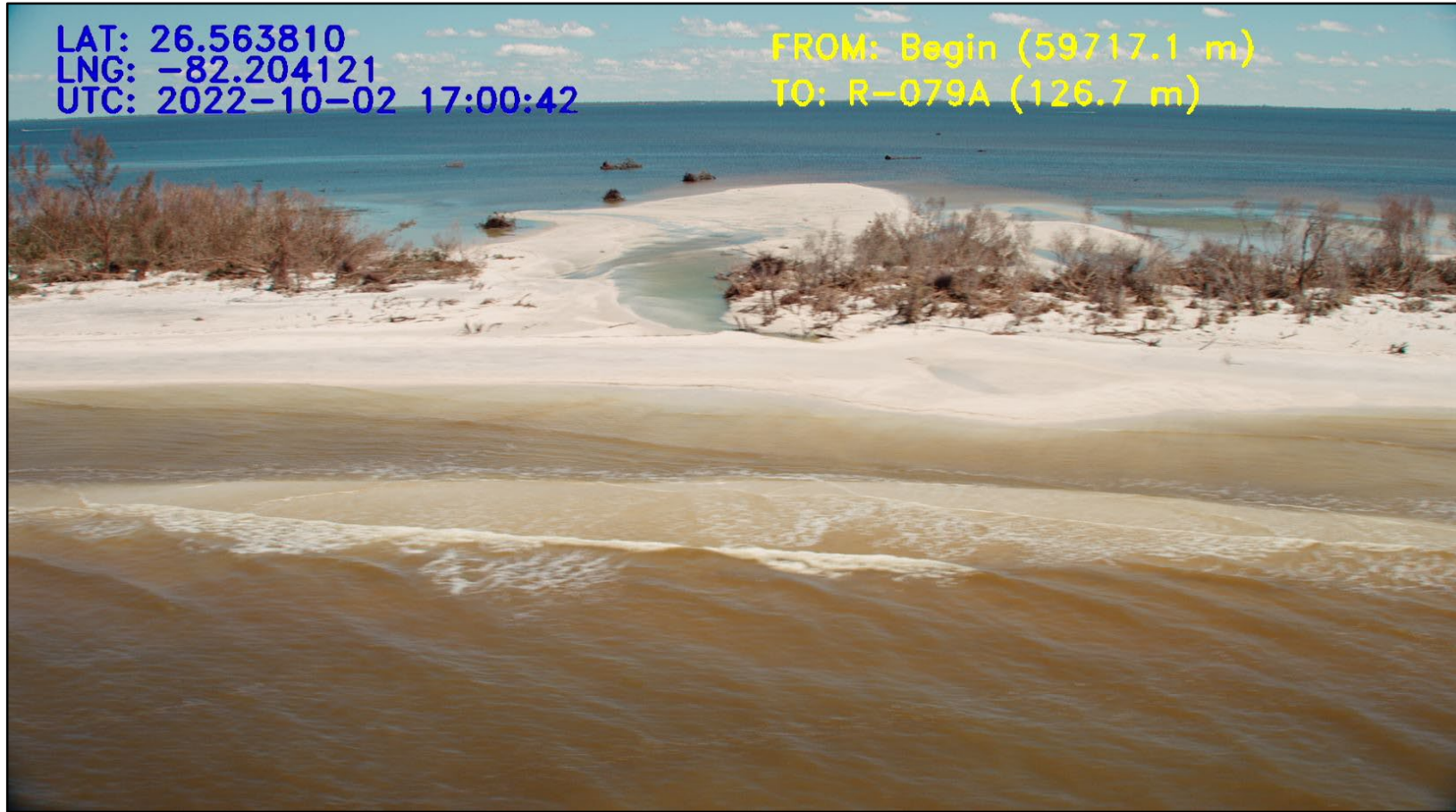
Hurricane Ian's beach and dune damages (Condition IV) on North Captiva Island (R-79) near Charley's Cut, video photo by Camera Copters and Active Camera Systems
