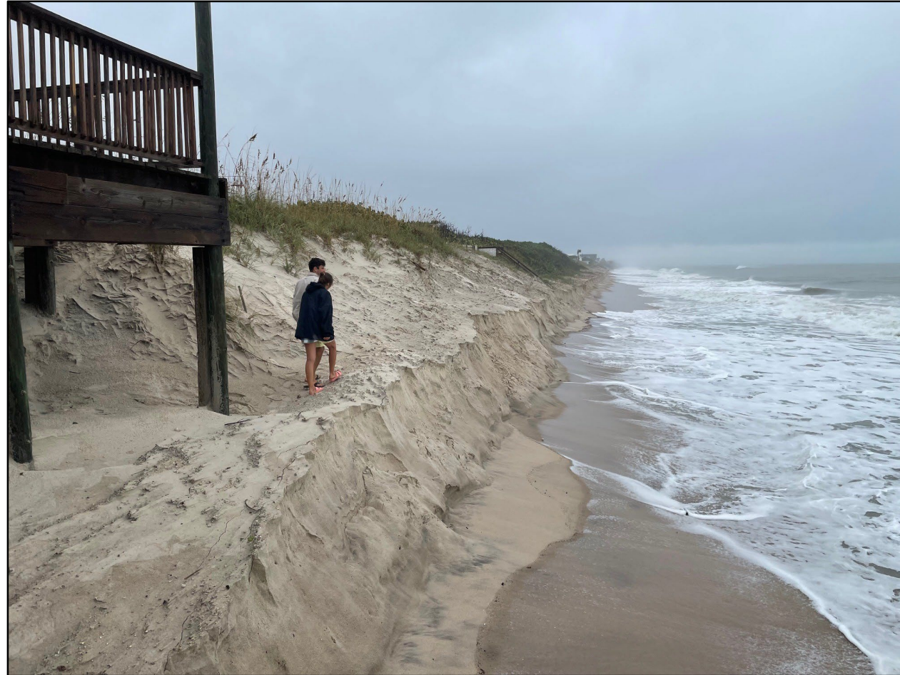
Major beach and dune erosion (condition IV) at South Beaches (Floridana) in Brevard County, near R-188
