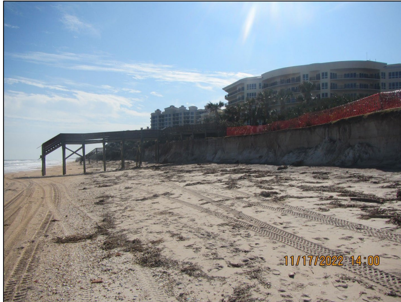
Major beach and dune erosion (condition IV) at Ocean Hammock, near R-37
