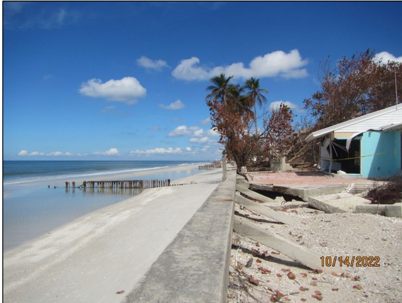
Naples beach with erosion condition IV, near R-85
