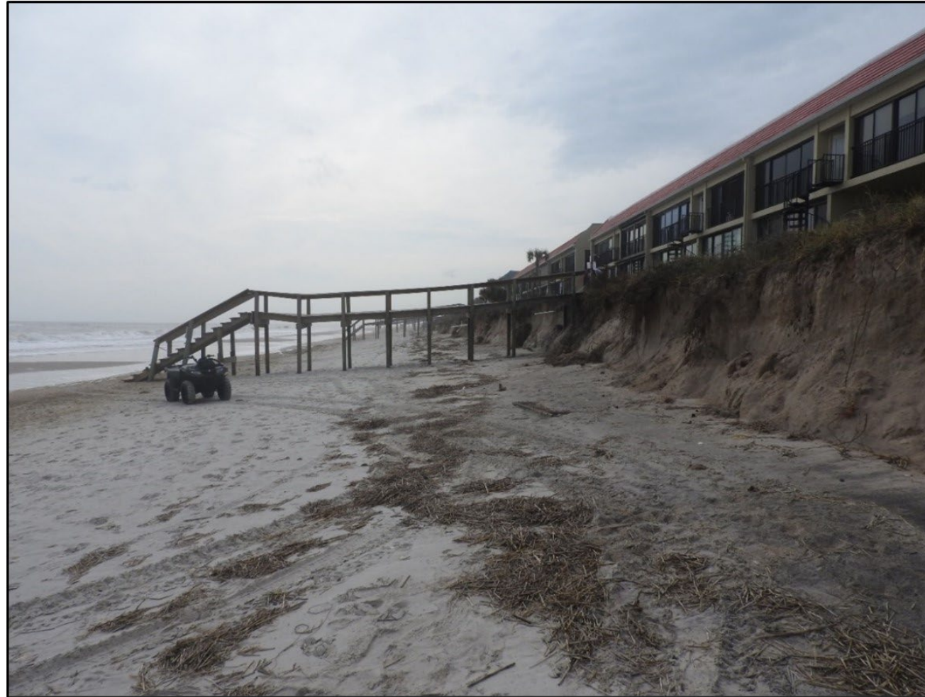
Major beach and dune erosion in Ponte Vedra Beach, erosion condition IV, near R-15
