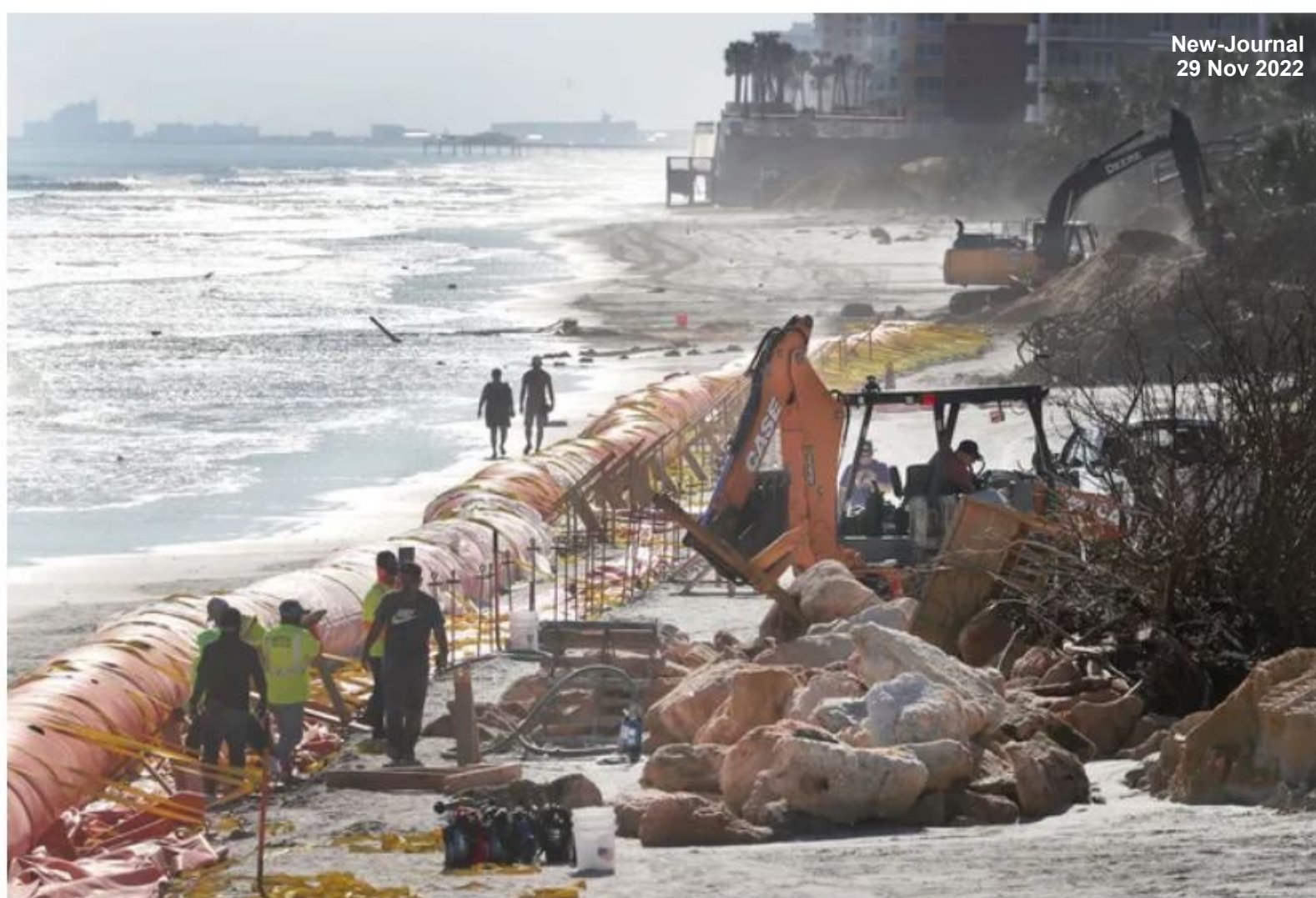
Construction crews install a Tiger Dam system Tuesday, Nov. 29, 2022, south of Frank Rendon Park in Daytona Beach Shores. The system is intended to offer a temporary protection against future erosion caused by storms. David Tucker/News-Journal
