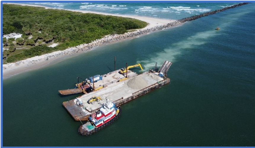
Figure 3: Fort Pierce Inlet Sand Trap (Phase I) Construction
