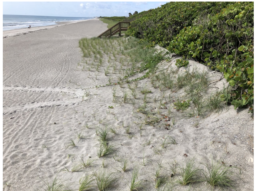
Vegetation, typically found on dunes, were planted on the newly constructed dunes along the Patrick Space Force Base segment. Credit: U.S. Army Corps of Engineers
