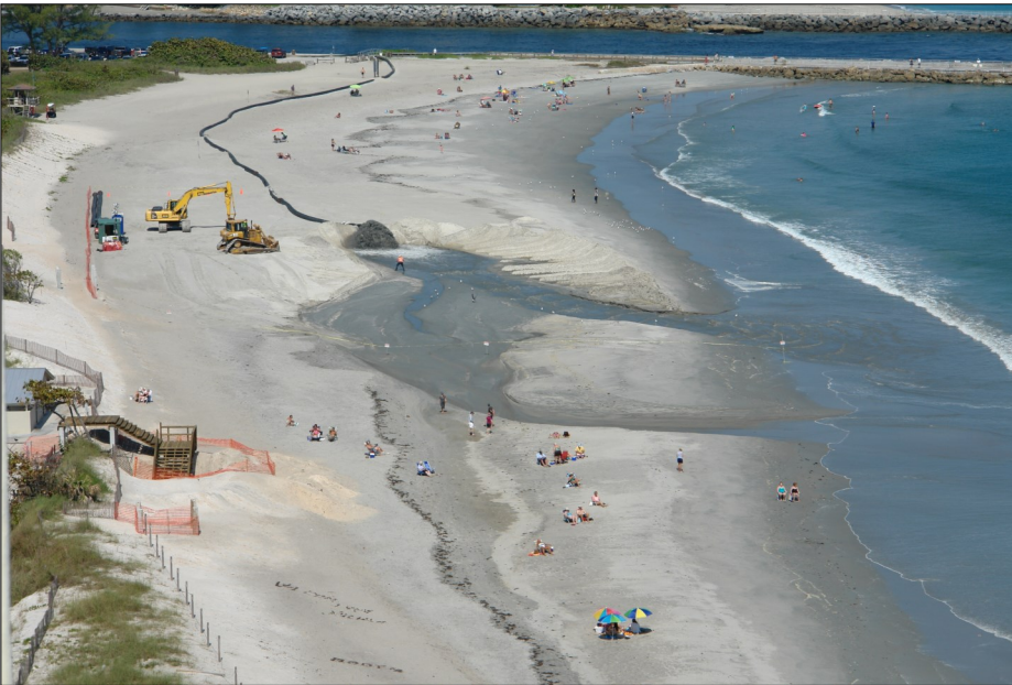
Samples being taken from the discharge slurry on the beach south of Jupiter Inlet
