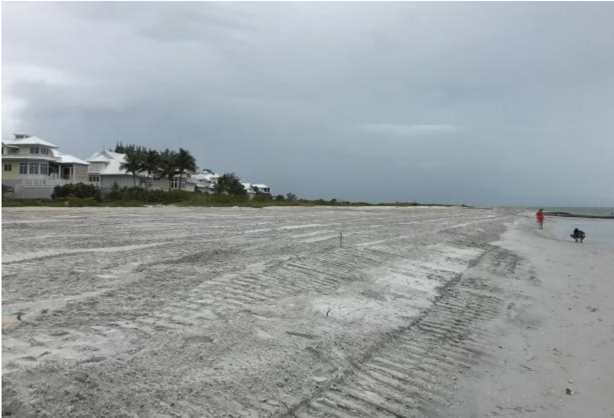
Figure 9. 2017 Project: View looking Southwest at Completed NBF.
