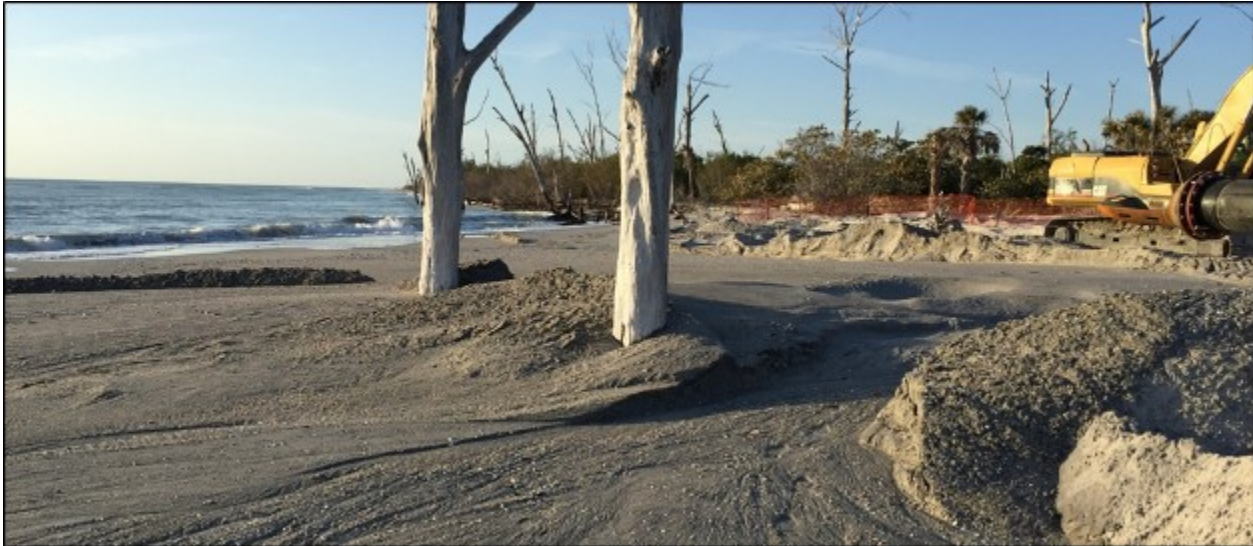
Figure 7. 2017 Project: View looking North at Starting Point of Beach Fill.
