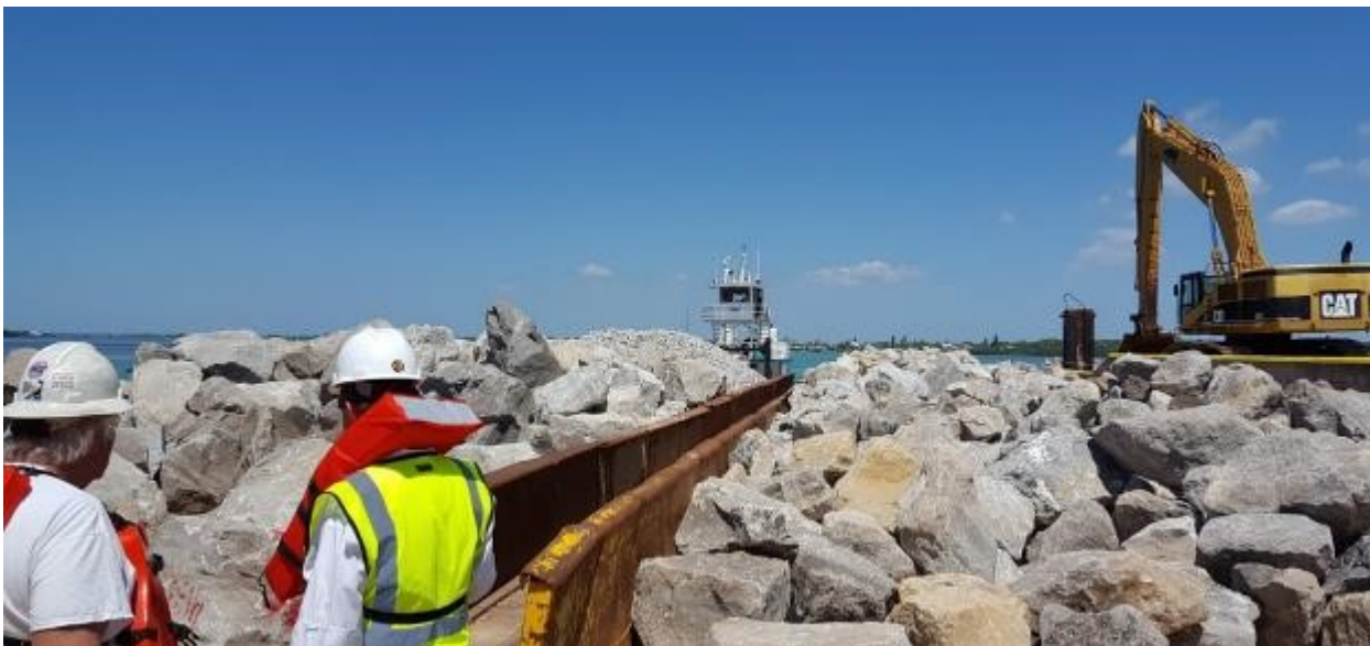
Figure 10. 2017 Project: Barges from Missouri Arrive with Bedding, Core, and Armor Stone.
