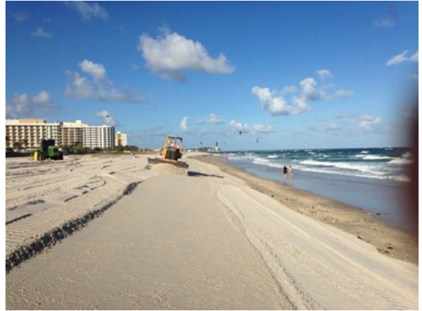
Photo of Broward County during previous Beach Renourishment (2014)
