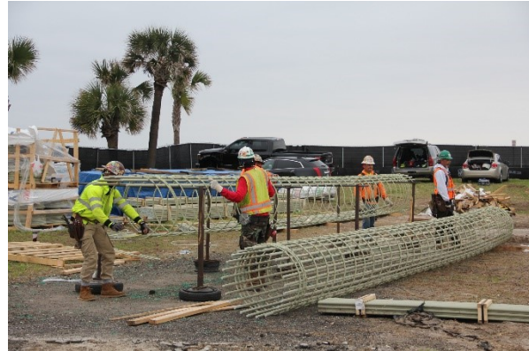
Figure 10: Installation of Continuous Spiral-Ties
