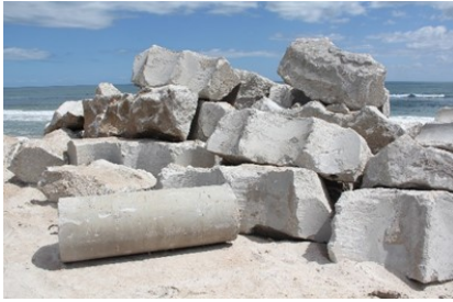
Figure 24. Guide-wall after removal
