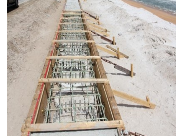
Figure 26: GFRP Pile-Cap rebar installation
