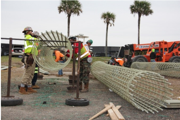
Figure 9: Assembly of GFRP secant-pile Cages
