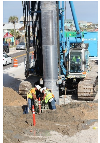
Figure 23: Cage Installed
