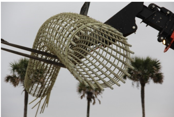
Figure 13: Lifting of GFRP Cage without "Toe"
