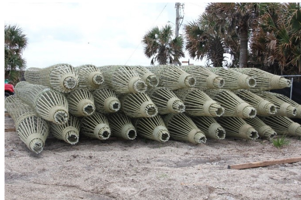
Figure 12: Storage of GFRP secant-pile Cages
