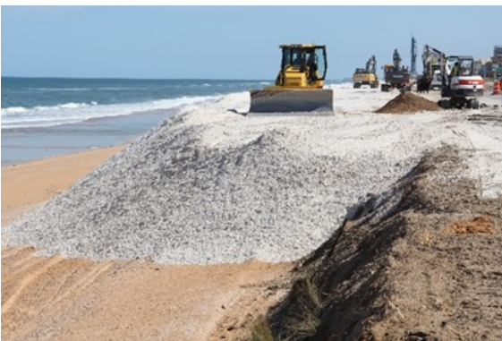
Figure 5: White sand, soil-backfill placement.
