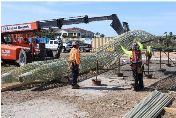
Figure 11: Lifting of GFRP secant-pile Cages
