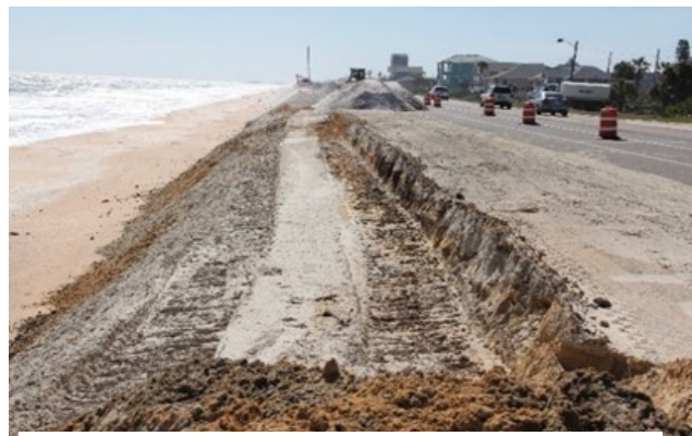
Figure 6: Backfill “cut-in” and step-down-profile.
