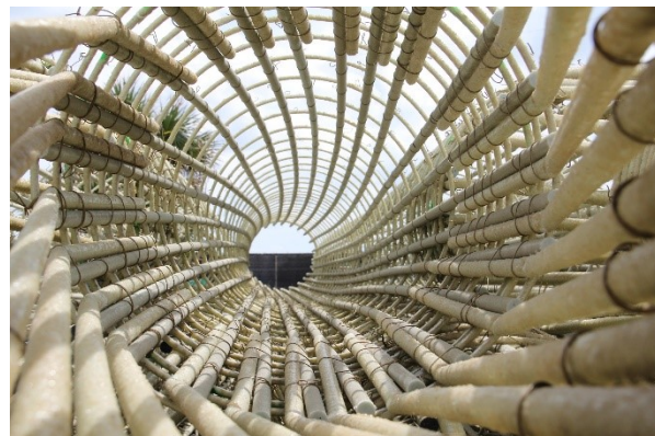
Figure 14: Inside View of GFRP secant-pile Cage
