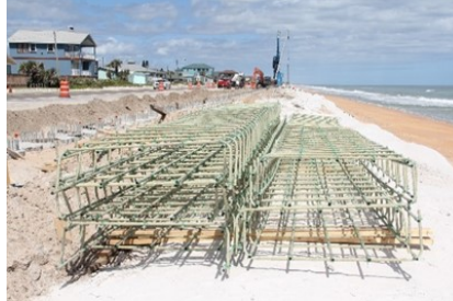
Figure 25: GFRP Pile-Cap rebar cage assemblies.
