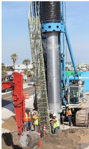
Figure 20: Cage Insertion
