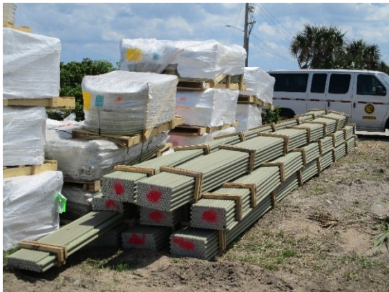
Figure 8: GFRP reinforcing delivery
