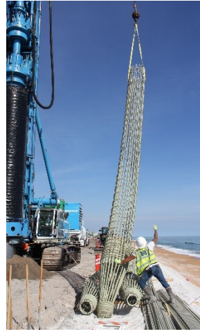
Figure 17: Pile Cage Lifting
