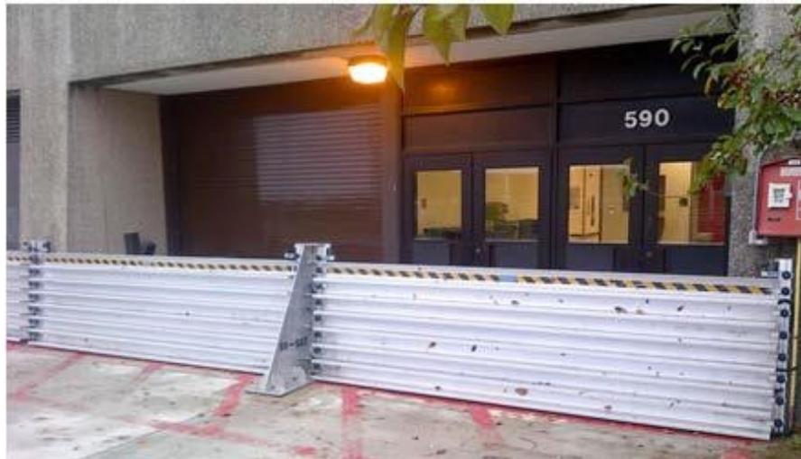
Temporary, Removable Door Dams at the U.S. Naval Academy in Annapolis, MD
