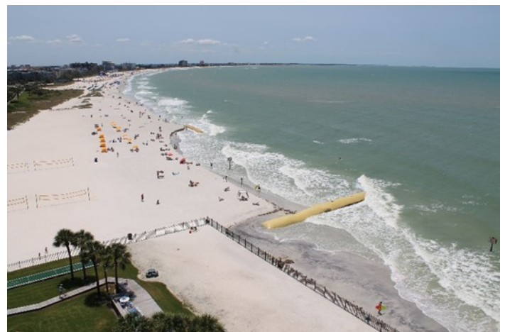
Figure 4. May 06, 2016 Post Geotextile tube removal.
