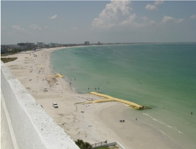
Figure 3. Photo approximately 2006 after the geotube groin construction is finished
