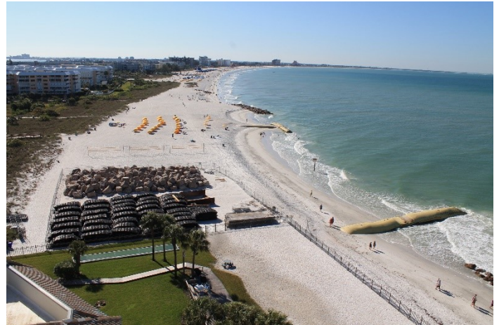
Figure 7. Southern 2 rock groins installed
