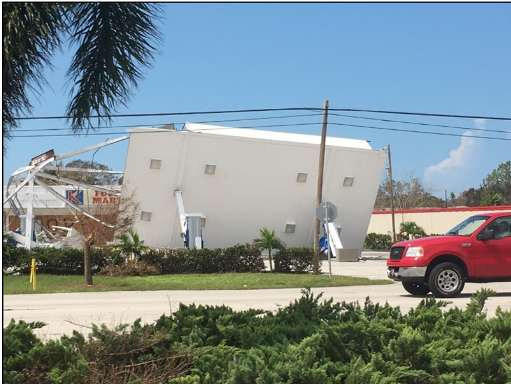
Damaged gas station in Collier County post-Hurricane Irma, September 2018
