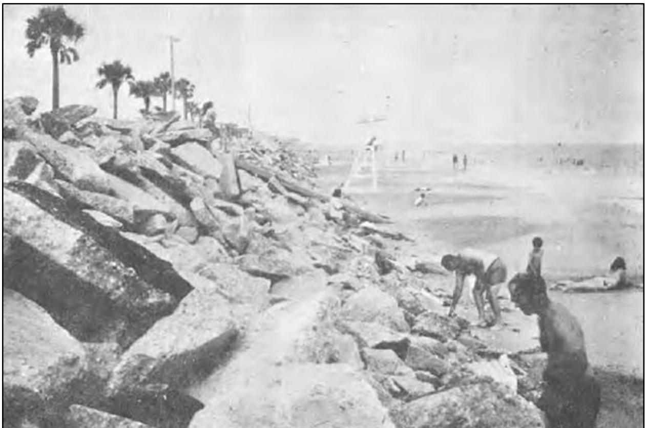
Figure 3: Fernandina Beach circa 1975. A large rock revetment protected the area behind it prior to the Federal Shore Protection Project.
