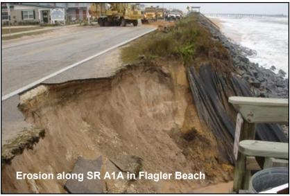
The recommended plan for Flagler County consists of a ten foot dune and beach profile extension along 2.6 miles of shoreline in Flagler Beach and mainly prevents damage to most vulnerable sections of State Road A1A, an important hurricane evacuation route. Initial construction will require approximately 330,000 cubic yards of sand, and each periodic nourishment event will require approximately 320,000 cubic yards. The renourishment interval is expected to be approximately 11 years, **Next Page**
