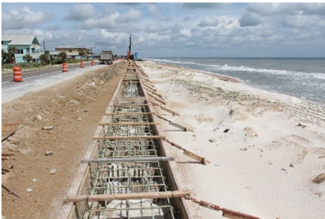
Figure 5 - "Cast-In-Place" Pile-Cap Formwork (June 2019)
