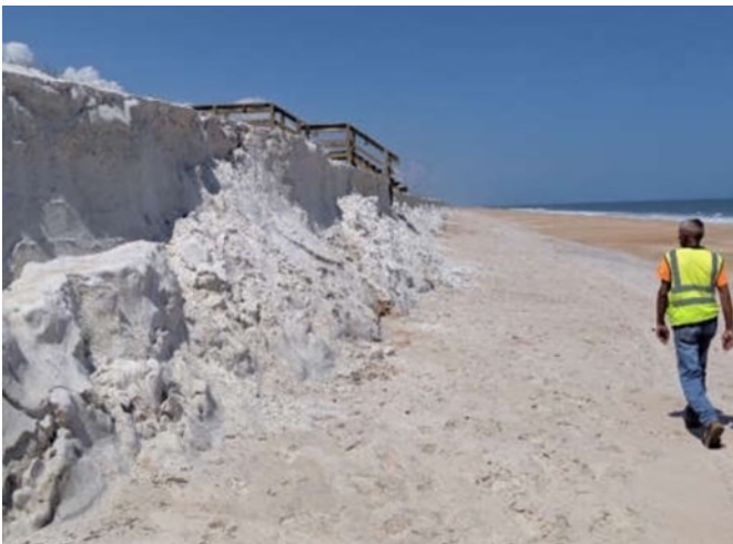
Figure 1 – Flagler Beach sand dune erosion post-Dorian (September 2019)
