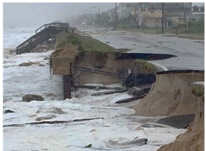
Figure 2 – Flagler Beach dune erosion and highway damage post-Matthew (October 2016)
