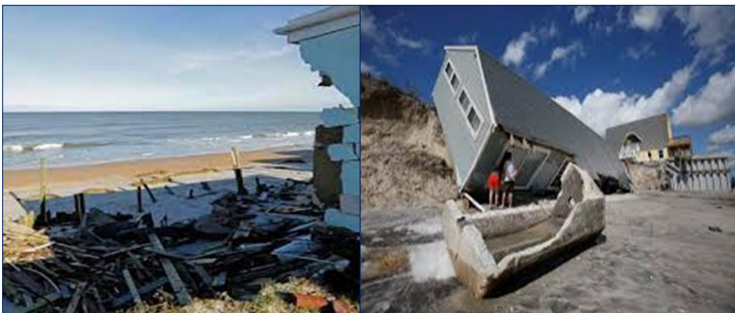
Photos of Damage from Hurricane Matthew 2016
