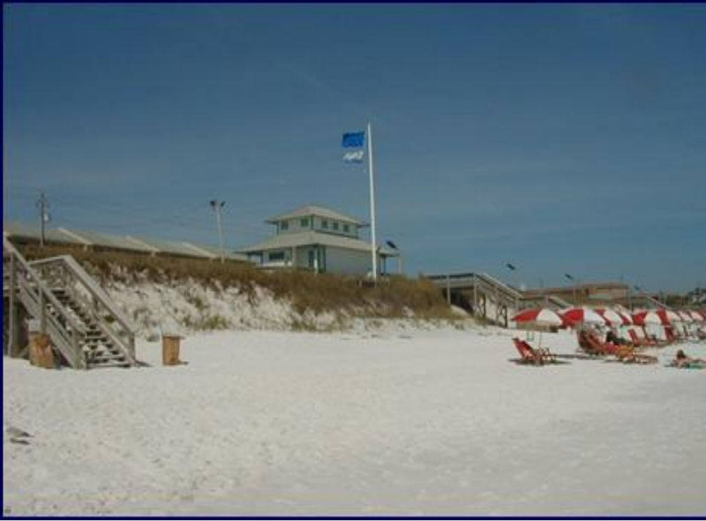
Pre-Hurricane Ivan photo of Miramar Beach Regional Beach Access restroom in western Walton County
