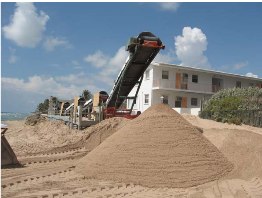
Conveyor systems placing sand on the beach
