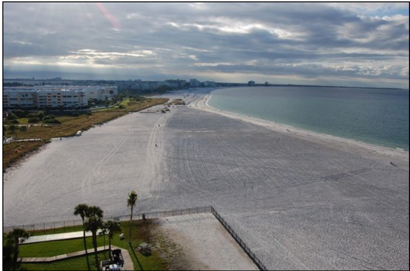
Upham Beach following construction
