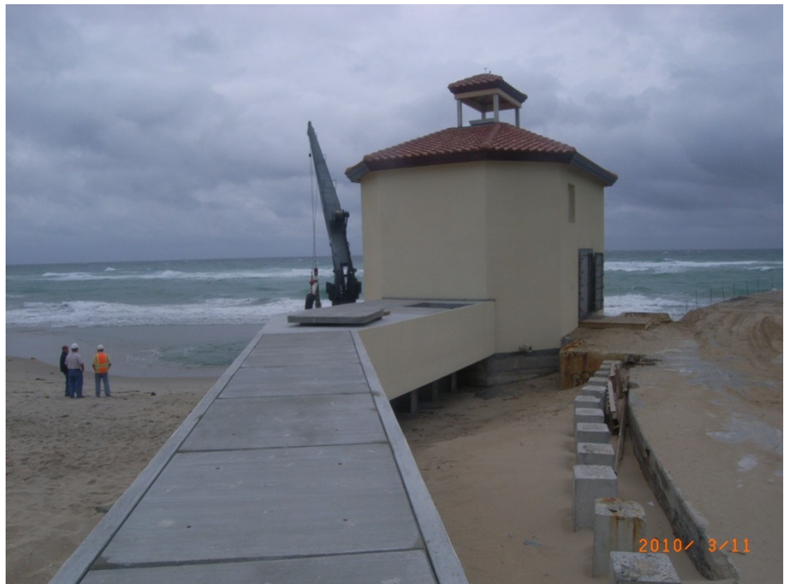
Reconstructed South Lake Worth Inlet Bypass Plant nearing completion
