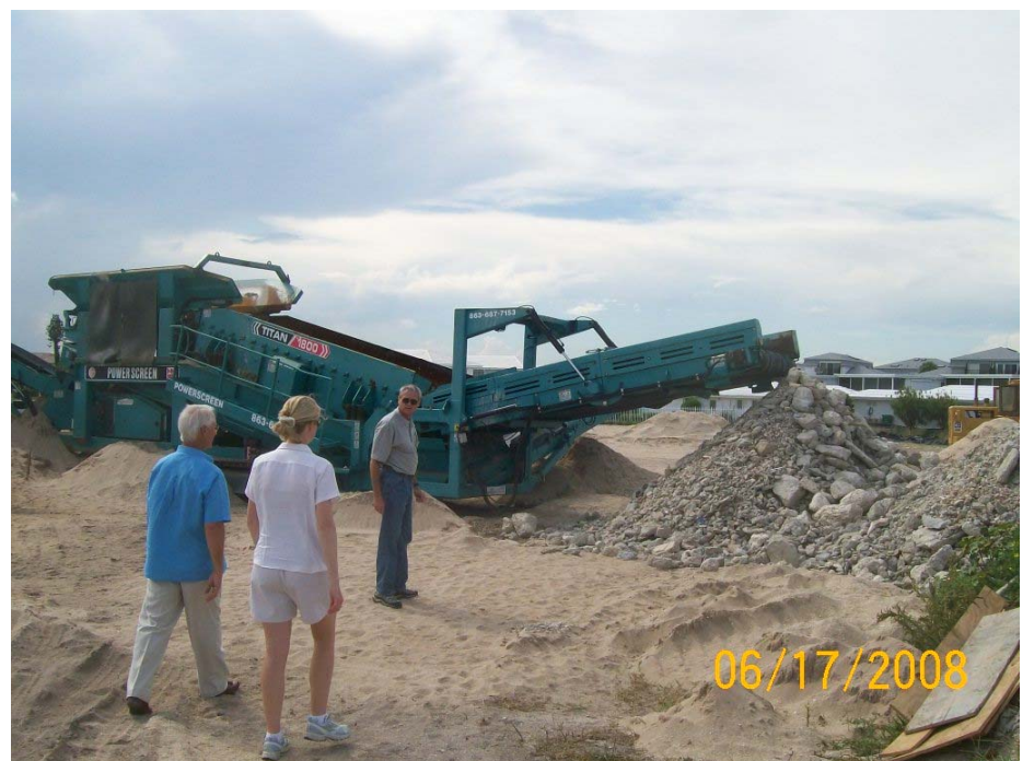
Sand screening operation for waste material at the stockpile location
